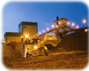
Avista's Kettle Falls Wood-Waste Generating Plant
