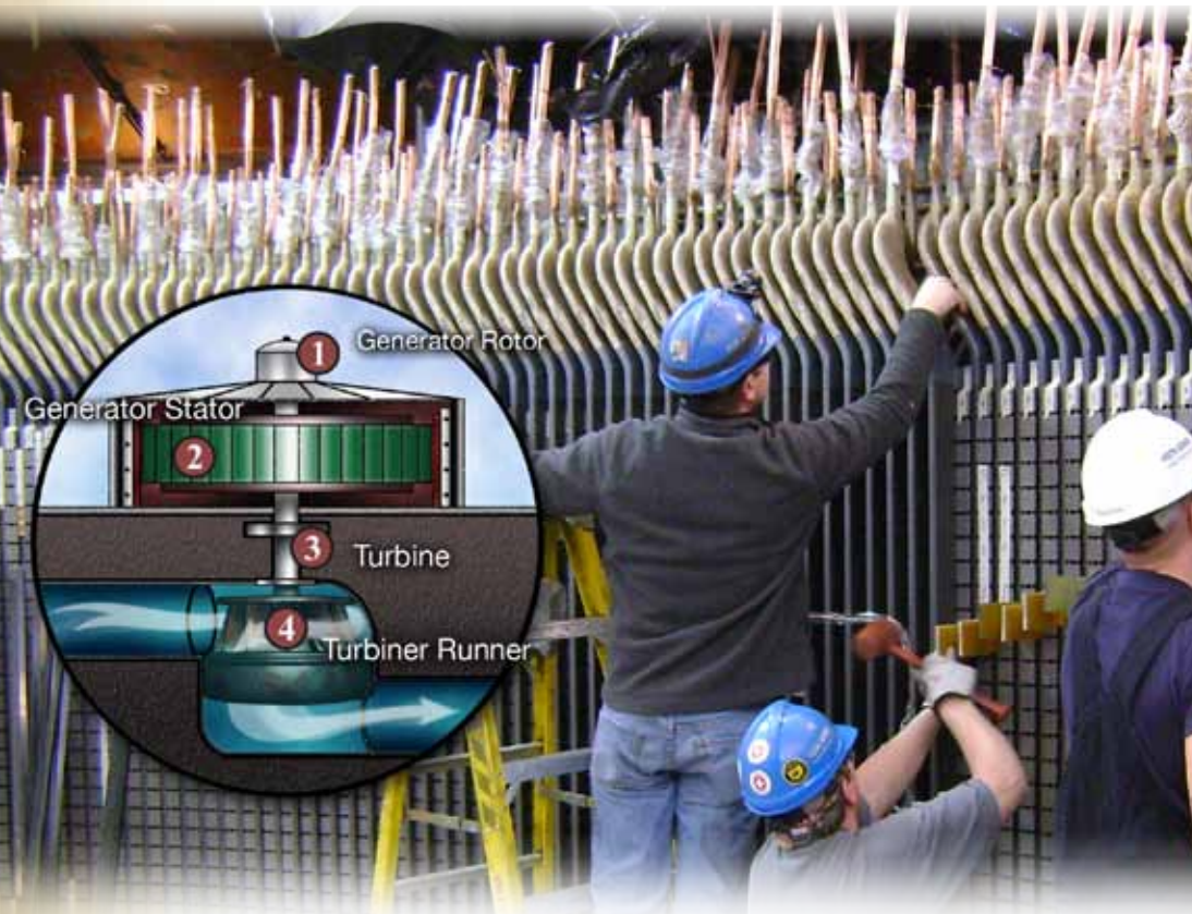
Workers rewind the stator of Unit 1 with new copper wire.
