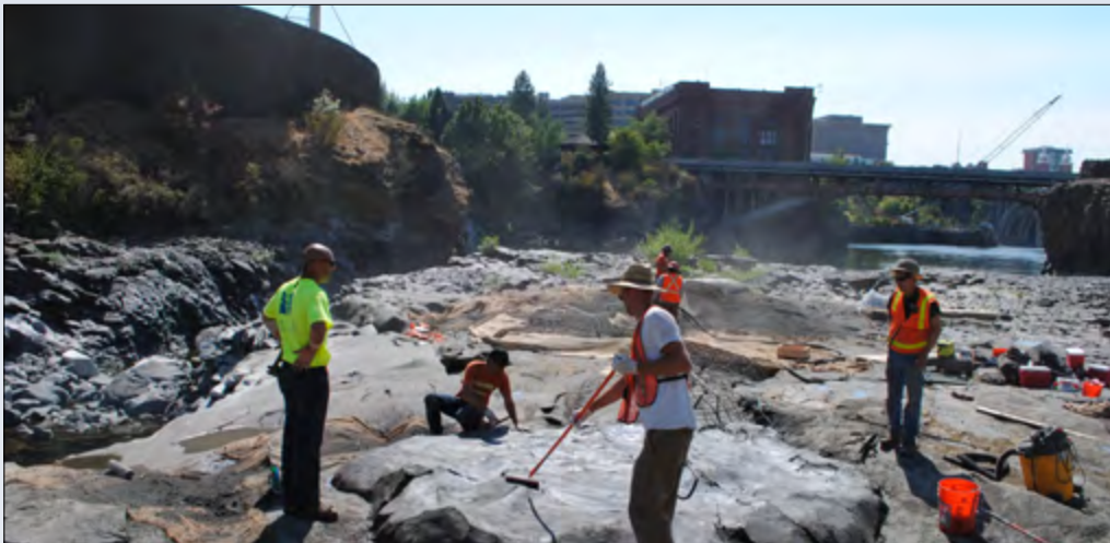
The Aesthetic Flows Project at Upper Falls Dam in downtown Spokane was completed. Beginning in the late 1800's, developers in Spokane cut into the bedrock to divert water during dry times. The Aesthetic Flows Project helps return the river's channels to a more natural state.
