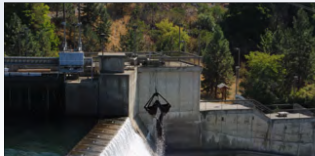
High river flows cause large amounts of rock, gravel and other materials to accumulate at the Monroe Street Dam. Removing the rock and placing it downstream helps keep the dams running efficiently and provides the material to support downstream habitat.
